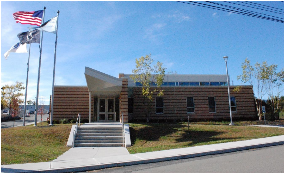
Image 1: North Shore Regional 911 Center
