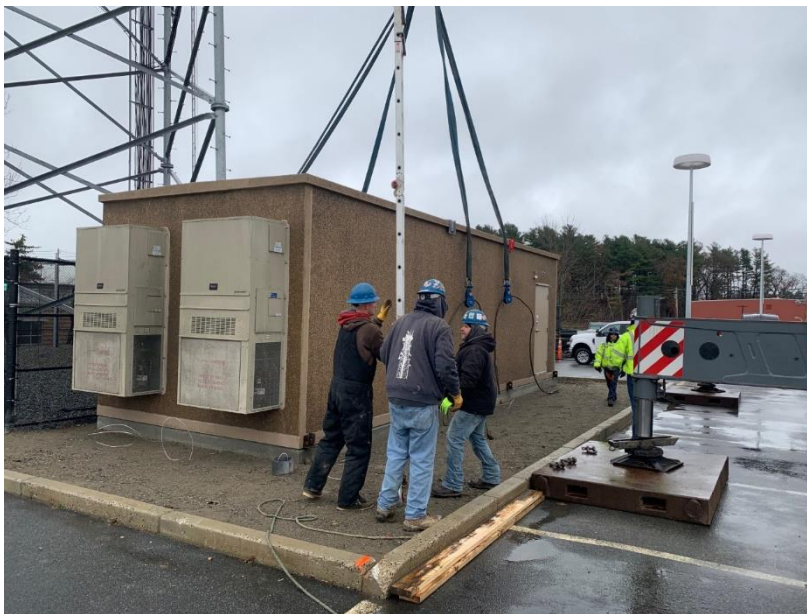
Image 16: Shelter placed on footing by crane
